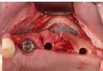
9. Intra-#25, #27 operative image. Incision and flap elevation. Removed healing abutment. Implant drilling at #25, #27. External sinus lifting.
